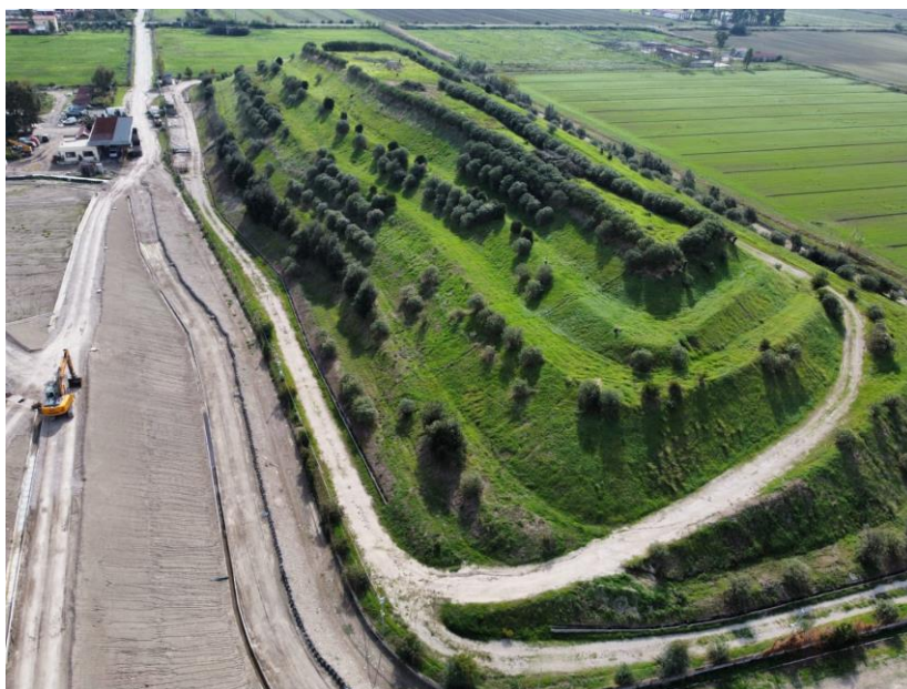
Figure 31: 3D view of the Bortolotto landfill - Aerial shot of 10/28/2021. You can observe the high grassing of the cap and the planting of numerous medium-sized trees.
