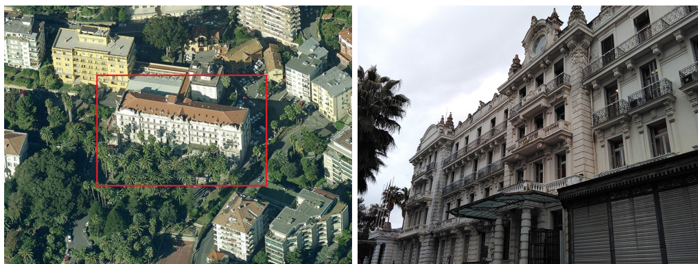
Figure A1: (a) Bird's-eye view of Bellevue Palace (from Bing Maps). (b) Front view of the building, showing the regular distribution of openings on the façade.
