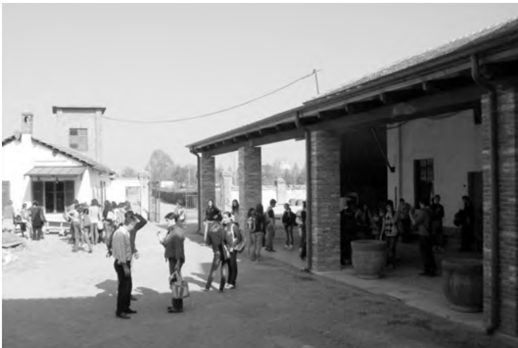
Figure 3-16 A group of students visit the renovated rice mill in Vercelli, Turin, Italy (Photo: by author)
