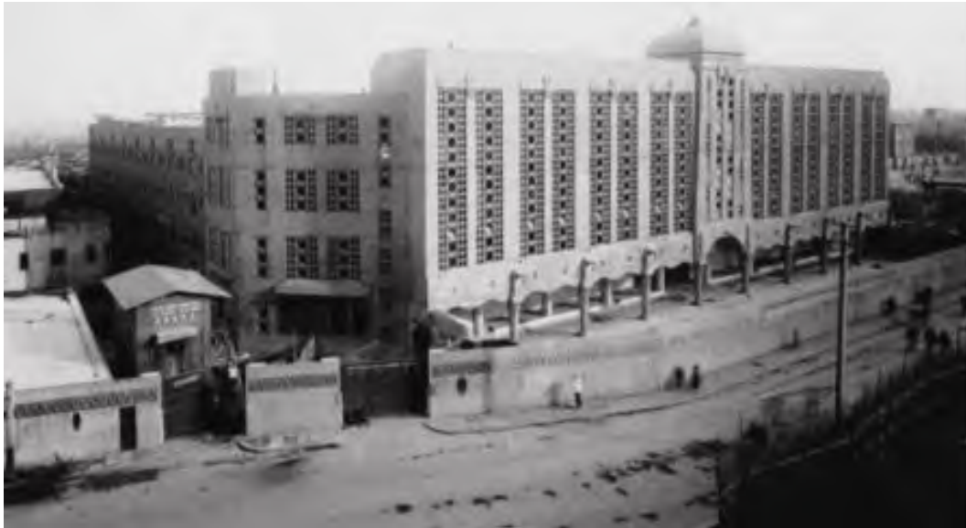
Figure 4-3 Shanghai Municipal Abattoir in 1937 (Source: Shanghai Municipal Archives.)
