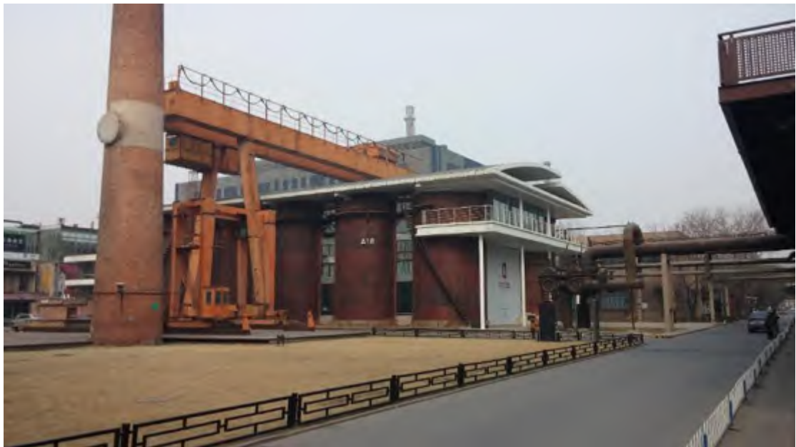
Figure 2-39 the industrial remains in Design-Park 751 in Beijing. The former gas plants was assessed as a Creative Industrial Agglomeration Area. (Photo: by author)
