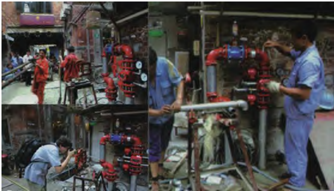
Figure 5-29 The renovation of fire control facilities ,2008 (Source: KE Xiongbin and others, “The Protection of Characteristic Streets in Modern City:A Case Study of Shanghai Tianzifang,” HUAZHONG ARCHITECTURE, 2011, 184–188.)
