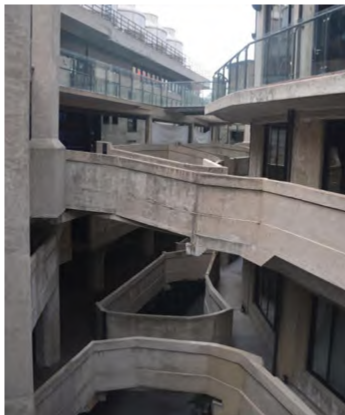
Figure 4-37 The cross- bridges after restoration, 1# building, 1933 Old Millfun (Photo: by author)
