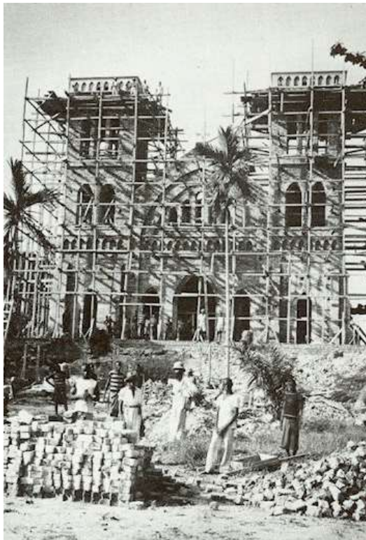
FIGURE 153: THIS COULD BE THE CONSTRUCTION OF THE CATHEDRAL SQUARE.
