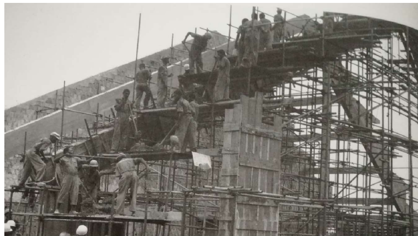
FIGURE 203: THE SCAFFOLDING OF SAINT AUGUSTIN REMAINS ONE OF THE MOST FAMOUS PICTURES OF PAUL DEQUEKER'S BUILDING SITES
