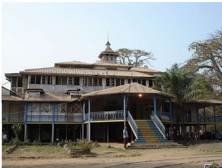
FIGURE 34 : FORMER RESIDENCE OF THE GOVERNOR GENERAL OF THE BELGIAN CONGO, IN BOMA . PHOTO: P. CLEMENT 2008.
