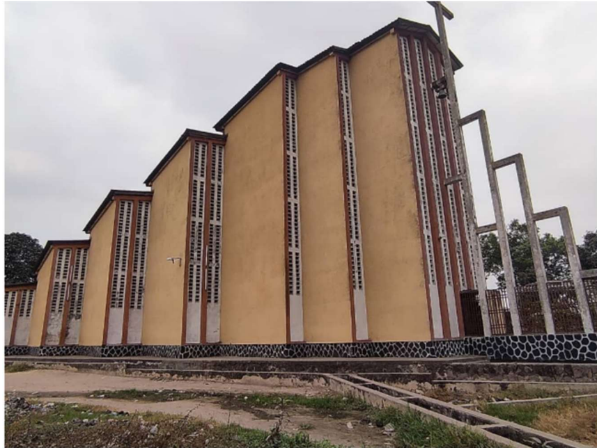
FIGURE 223: CONTRARY TO THE ORIGINAL IDEA OF THE ARCHITECT PAUL DEQUEKER, WHO USED UNPAINTED WALLS, THE WALLS ARE NOW PAINTED. PHOTO: VICTOR BAY 2021
