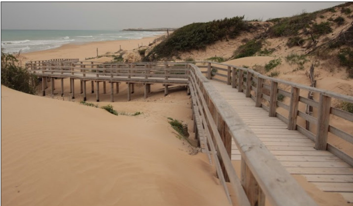
Fig. 36 – Boardwalk built on the dune ridge of Punta Braccetto. The picture has taken in 2016.
