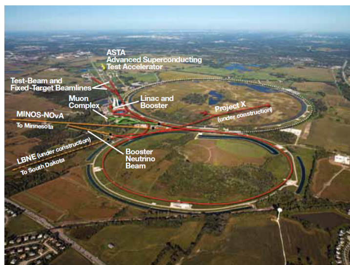
Figure 1.2: Aerial view of the Tevatron at Fermilab, that is an example of circular accelerator
