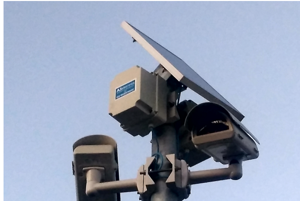
Figure 4.11: Picture showing the final field test installation.
