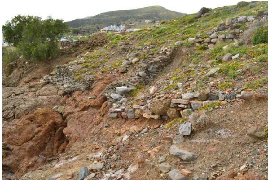
Fig. 34 Retaining walls on cape Psamidouri.
