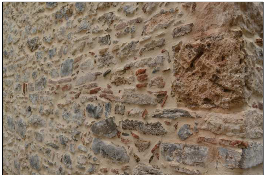
Fig. 68 Aghios Georgios chapel masonry, embedded marble block.
