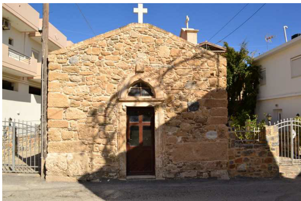
Fig. 98 Masonry of Panaghia chapel, embedded stone and marble blocks.
