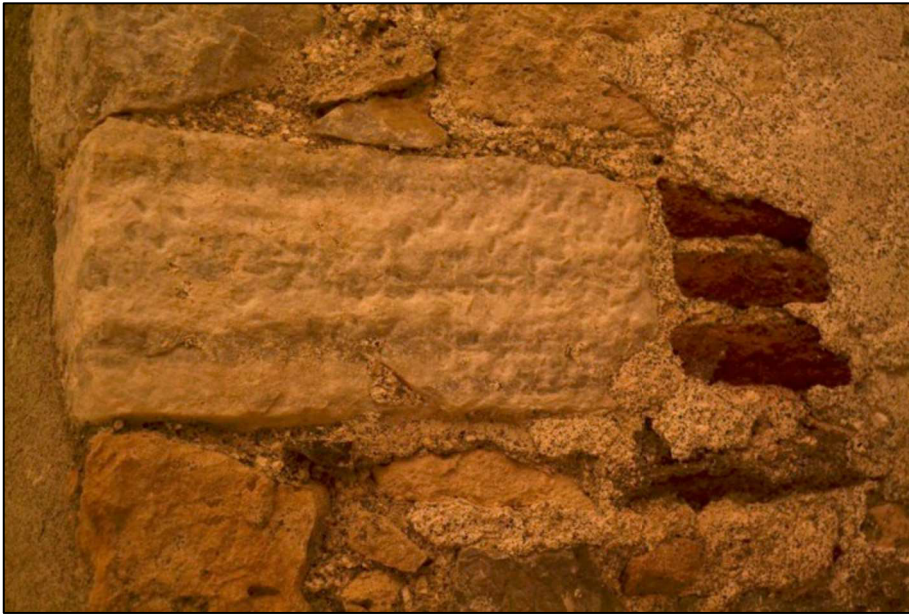
Fig. 68 Aghios Georgios chapel masonry, embedded marble block.
