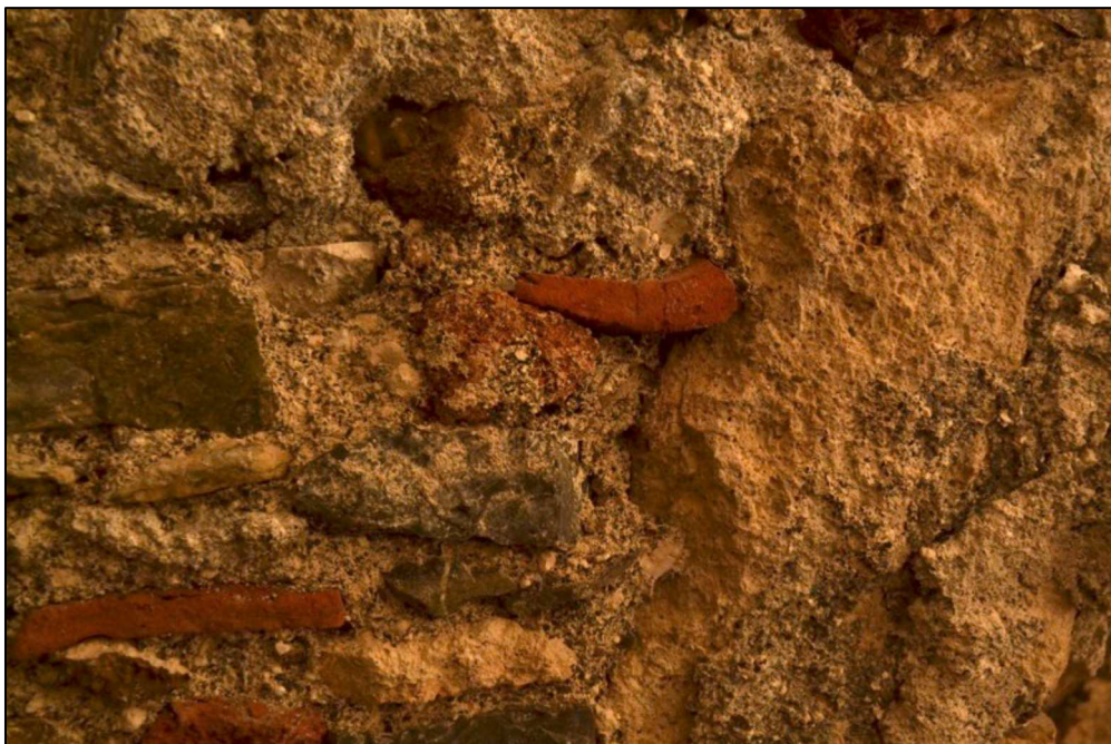
Fig. 69 Aghios Georgios chapel masonry, embedded tiles and pottery shreds.
