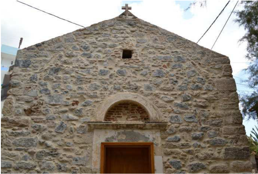
Fig. 71 Aghios Georgios chapel masonry, embedded tiles and stone blocks.
