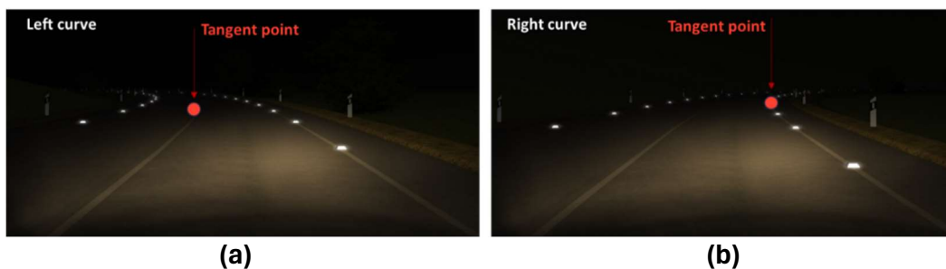
Figure 1. Road stud layout adopted in Portera et al. (2023). Assuming the tangent point mechanism is used (Land & Lee, 1994), in the case of a left turn (a) the gaze is directed toward a road sign without LED studs, which is in contrast with the case for right turn (b).
