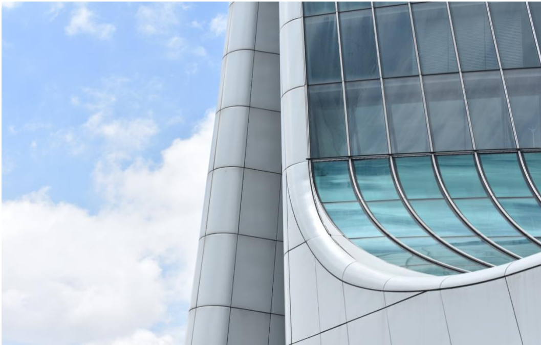
Figure 24: Generali tower façade, Milan
