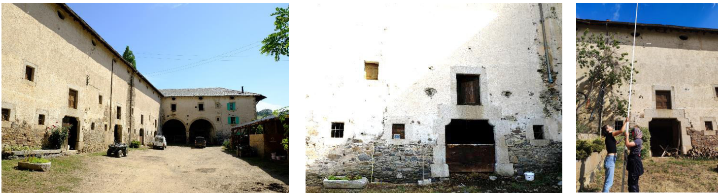
Figure 52: The northern complex, right: view from West of the inner court. Bizzarri, 2022. Centre: one of the main granite portals for the stalls, see also the granite frames for the windows. Bizzarri, 2022. Left: Giulia Bizzarri and Claire Larroque by the photographic/photogrammetric recording of the building. Rendu, 2022.
