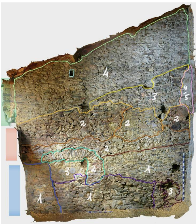
Figure 51: Overview of the inner western façade by the Building CF2 of the Southern Complex. The lower section can be seen as belonging to a first phase of construction (1- blue), possibly tied to the preceding structure in the area or the connection with Building CF3. The presence of a number of broken and slightly collapsing sections hint at the previous presence of structures attached to the wall that are no longer visible – possibly a manger. Phase 2 (red-yellow) involves the construction of the arched structure in the southern section of the façade, and the masonry units above. The holes present on the higher end of this part of the façade hint at the presence of a roofing structure that used to be placed below the current one. Also, the roofing structure seems to have followed a two-slopes rather than being the one-slope roof visible today. Phase 3 (yellow-green) is connected to the modification of the masonry structure right above the second phase and possibly the dismantling of the structure connected to the arch placed below, with its filling through rubble and other fragments and materials. Phase 4 is the highest section of the wall, tied to CF3. Photo: Bizzarri, 2022. Photogrammetric elaboration and notes: Bizzarri, 2023.
