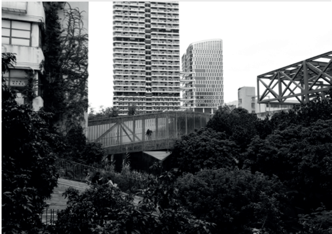
Figure 4.19_OCT-Loft: the creative area and the real estate developments surrounding the former industrial site. On the right, the B10 Building renovation in progress. Picture by the author.
