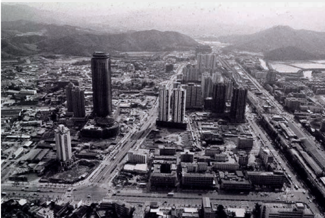
Figure 2.5 The centre of Luohu under construction in 1981, with Shenzhen’s original landmark building, the Guomao (International Trade). The construction of Guomao gave origin to the expression “Shenzhen Speed” and it was a destination for Deng Xiaoping on his 1992 Southern Tour. Source: South China Morning Post.
