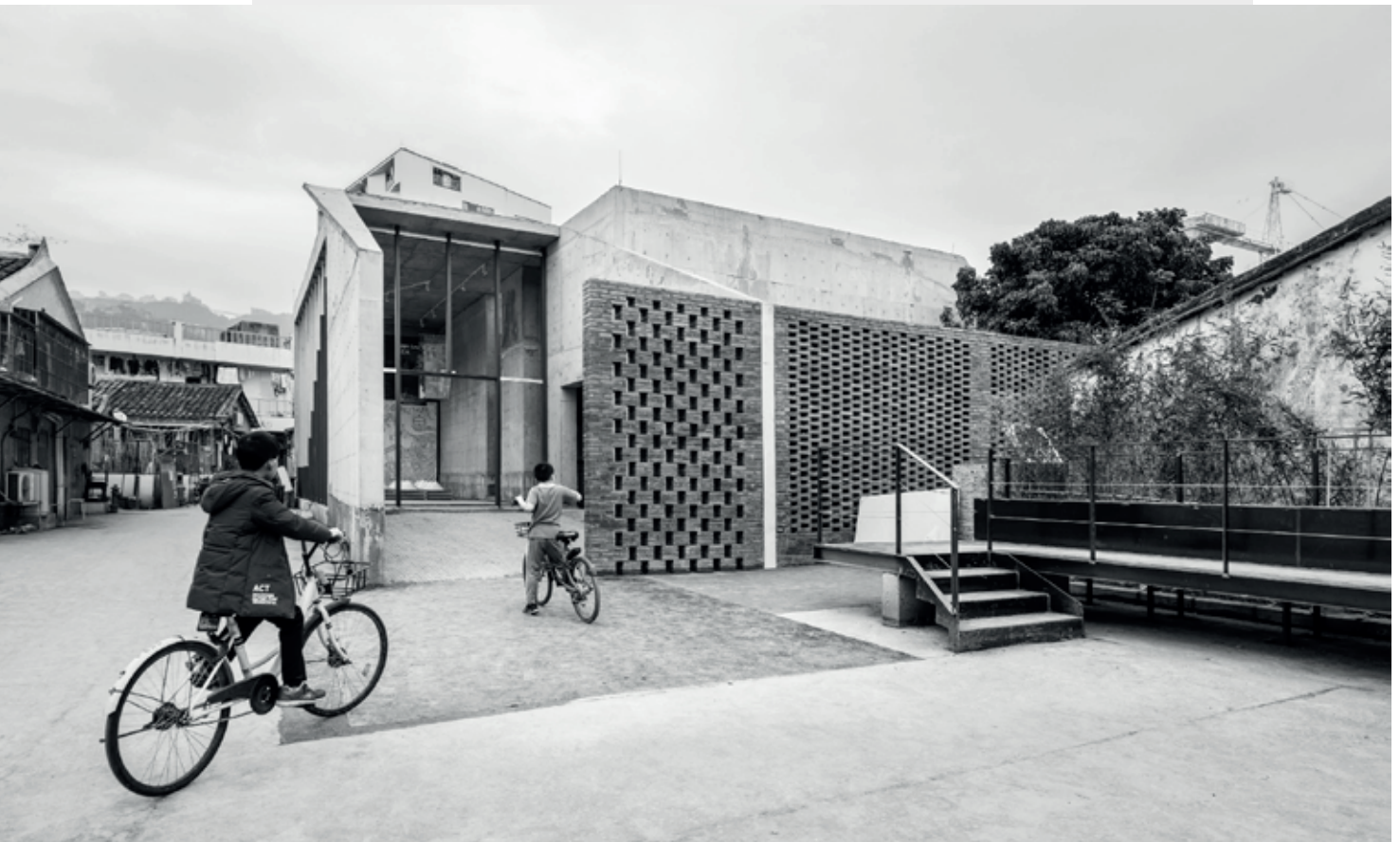
Figure 5.42_2017 Shenzhen Biennale renovation plan: the Dameisha Exhibition Hall and the “Glowing Square” designed by NODE. © NODE.
