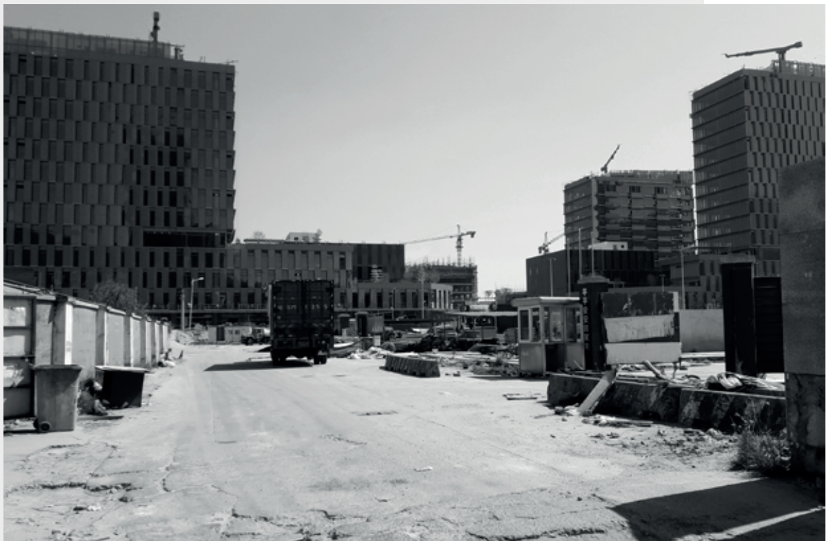
Figure 4.49 Building site of the Prince Bay development. Picture by the author.
