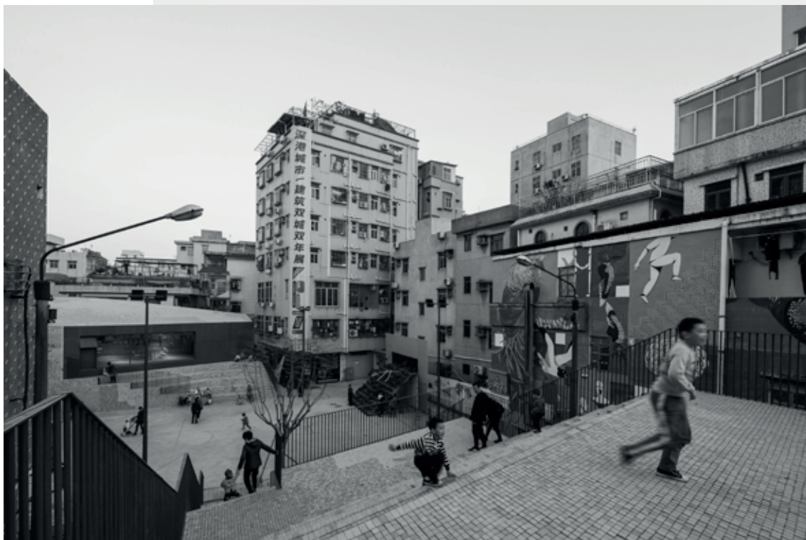
Figure 5.13_Baode Square area after the 2017 Shenzhen Biennale transformation: the basket court and the playground, the building B4 in the background. Picture by Zhang Chao. Source: Shenzhen Biennale of Urbanism\Architecture Organizing Committee archives. © Shenzhen Biennale of Urbanism\Architecture Organizing Committee.
