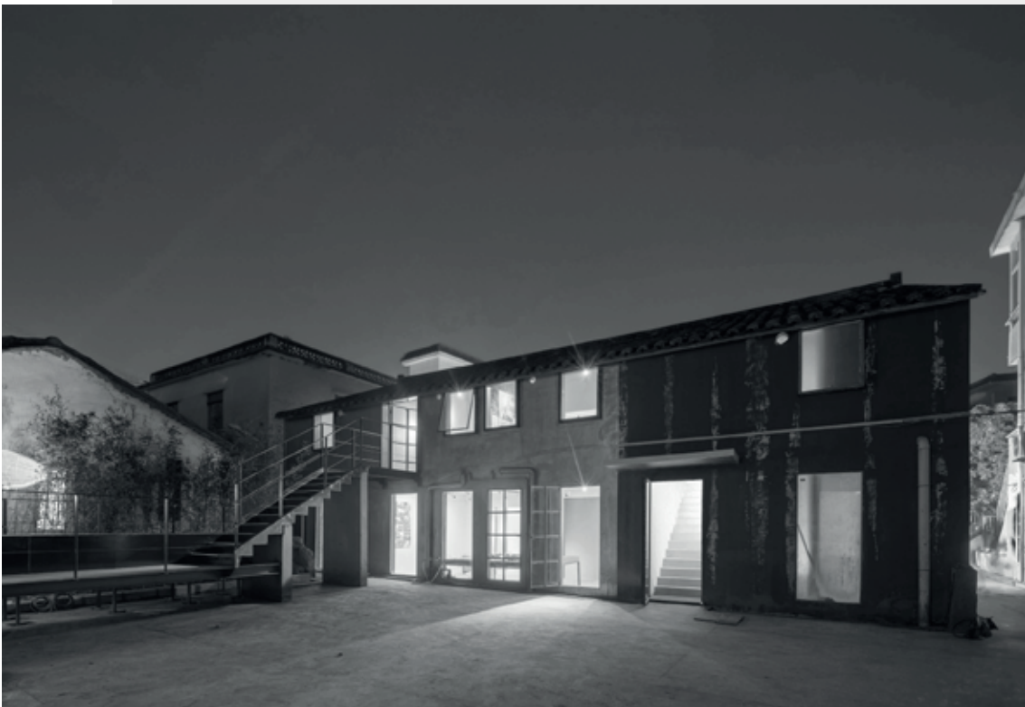
Figure 5.40 2017 Shenzhen Biennale renovation plan: House no.9 transformation by NODE. © NODE.
