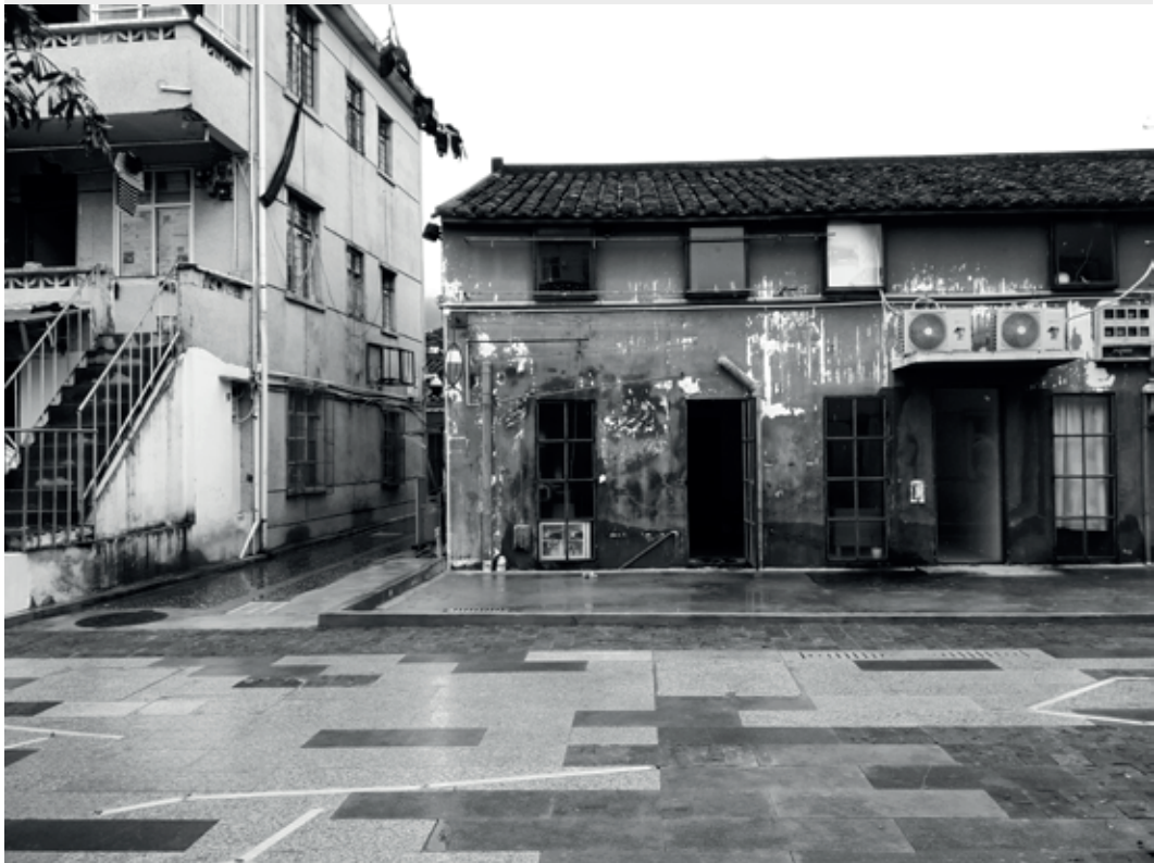
Figure 5.48_House no.9 unused after the 2017 Shenzhen Biennale. Picture by the author.
