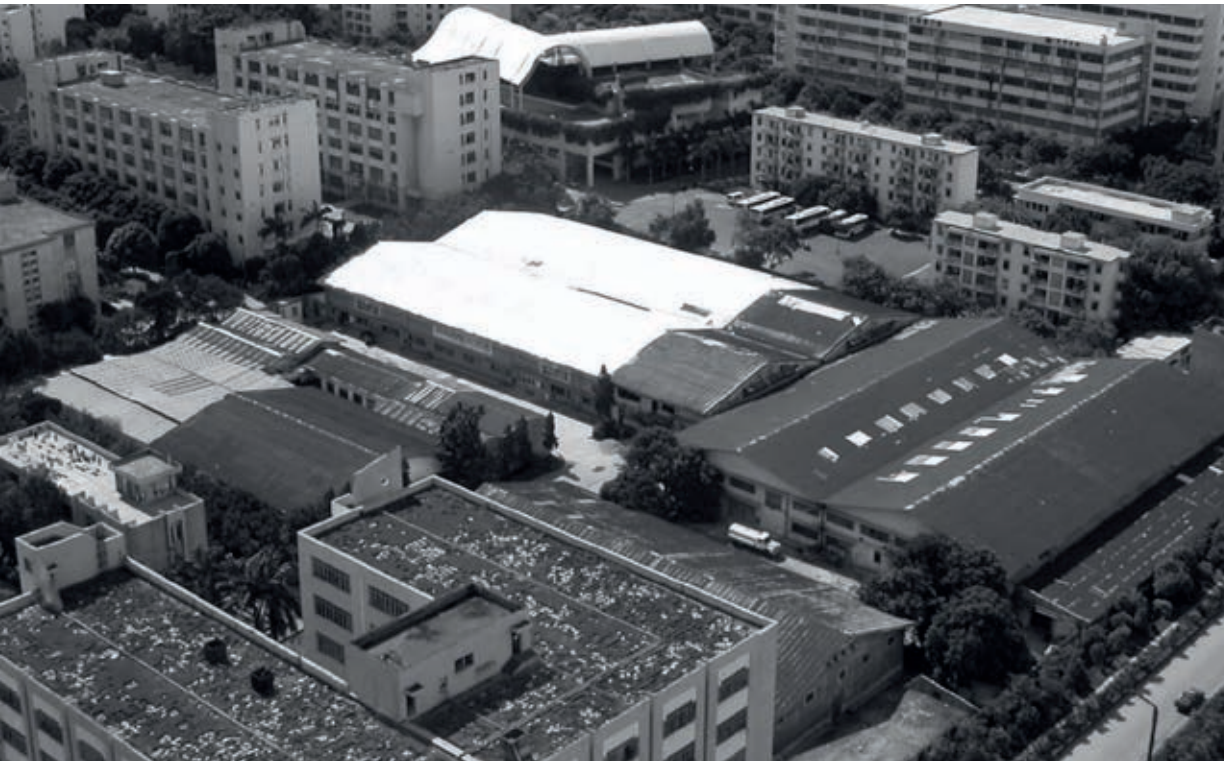
Figure 4.2_Overview of the Huaqiaocheng Eastern Area before transformation. Source: Shenzhen Biennale of Urbanism\Architecture Organizing Committee archives. ©Shenzhen Biennale of Urbanism\Architecture Organizing Committee.
