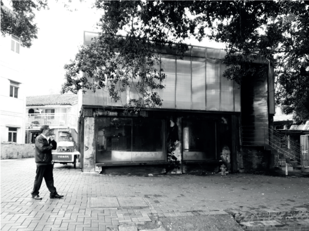
Figure 5.47_House no.10 unused after the 2017 Shenzhen Biennale. Picture by the author.
