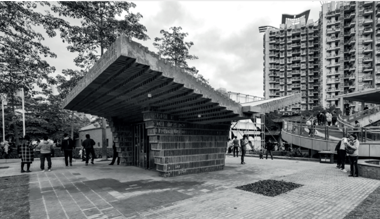
Figure 5.9 The concrete, brick and glass information pavilion designed by Yung Ho Chang (Atelier FCJZ) at the Southern entrance of Nantou Old Town. Source: Shenzhen Biennale of Urbanism\Architecture Organizing Committee archives. © Shenzhen Biennale of Urbanism\Architecture Organizing Committee.
