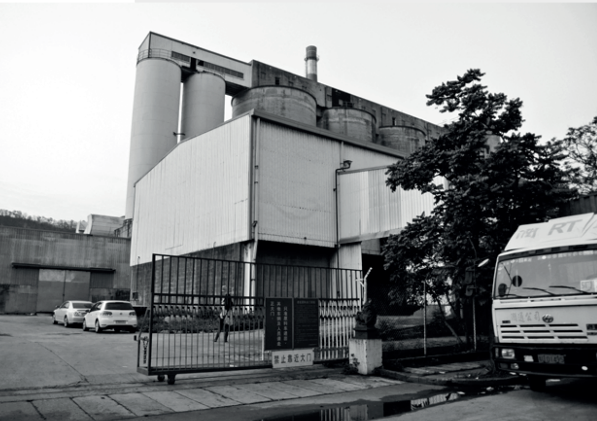
Figure 4.22_The Guangdong Float Glass Factory before the transformation: site entrance. Source: O-Office Architects. © O-Office Architects.
