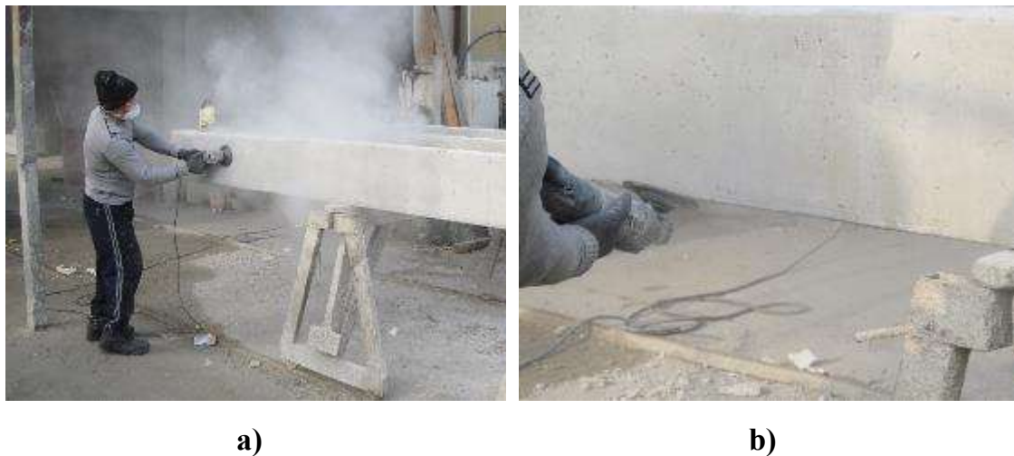
Figure 3-4 Surface preparation: a) mechanical grinding; b) rounding of the corners
