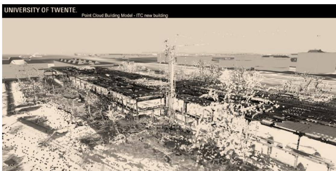
Figure 28. The VR web navigation (PCBM model) of the new ITC building (La Guardia et al., 2022b).
