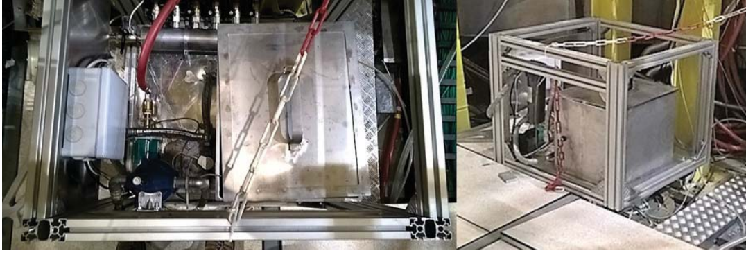
FIGURE 7.62: Left: Top view of the cooling system; Right: the cooling setup. Both the picture is for the bottom part
