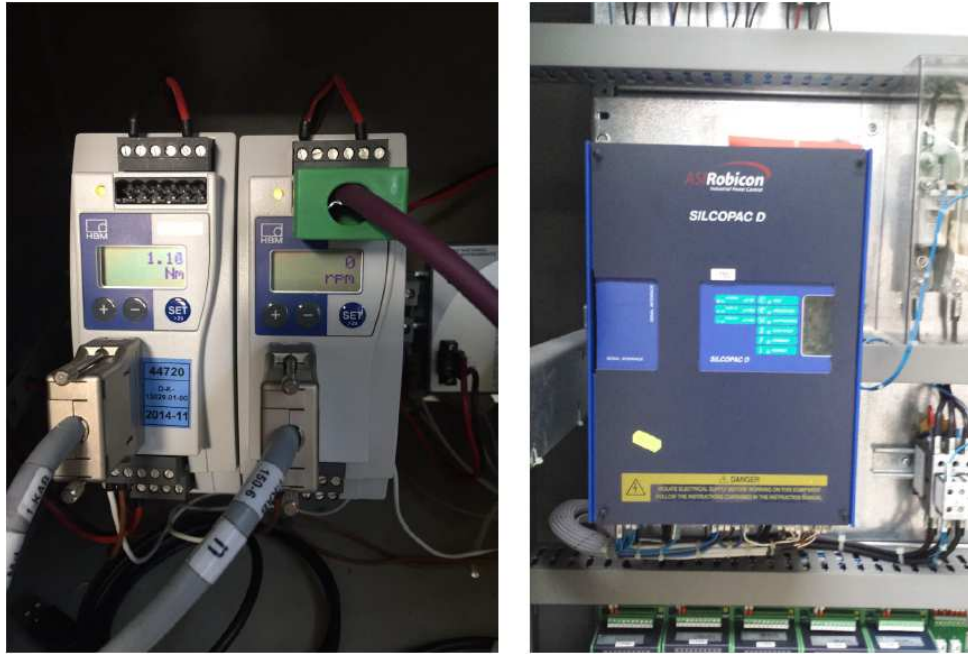
FIGURE 3.11: HBM MP60 signal conditioners for torque and rotational speed signals (left) and AC/DC converter Ansaldo Silcopac D (right).
