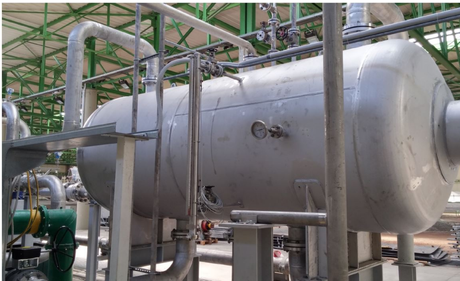
FIGURE 3.3: View of the Tank.
