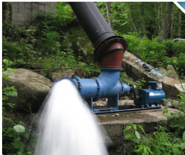
FIGURE 2.3: Example of an axial PAT for rural electrification [27].
