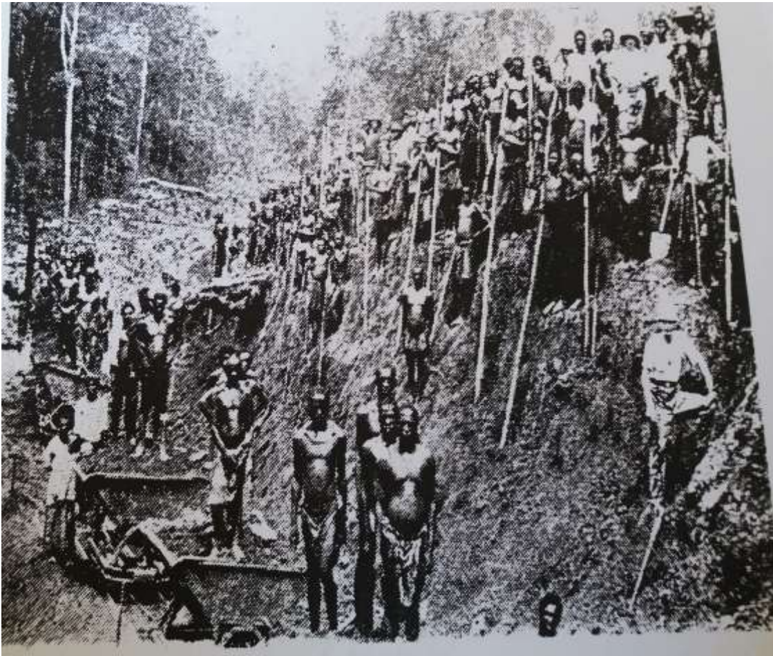
Figure 3: Failed Track Laying of the Northern Line Railroad
