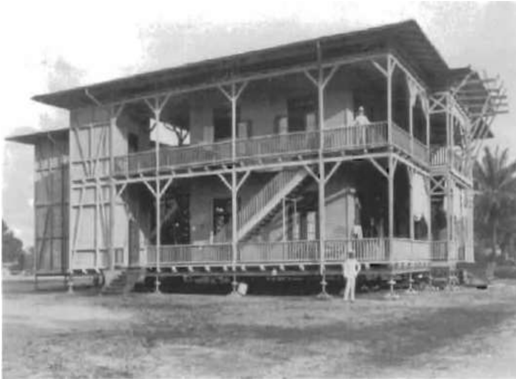
Figure 10 : Prefabricated House Presented at the Berlin Exhibition in 1896 and Reassembled in Douala
