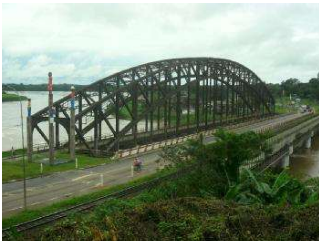
Figure 4: German Iron-bridge on the Sanaga River
