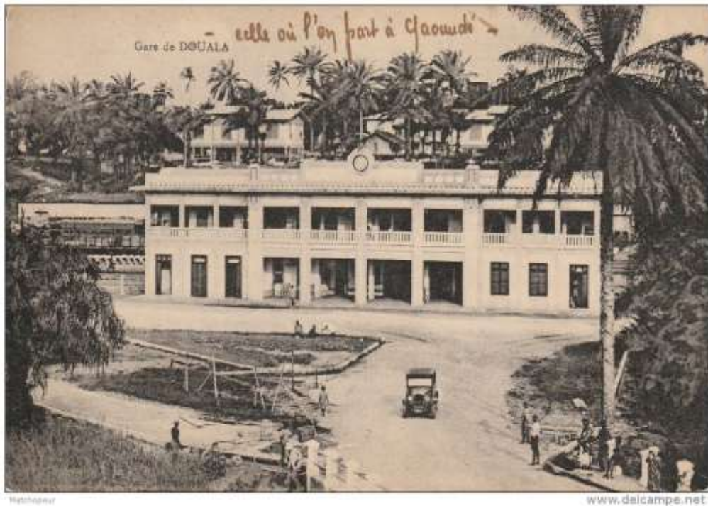
Figure 26 : The Last Rail Station at Besseke (Douala), Destroyed in the 1980s
