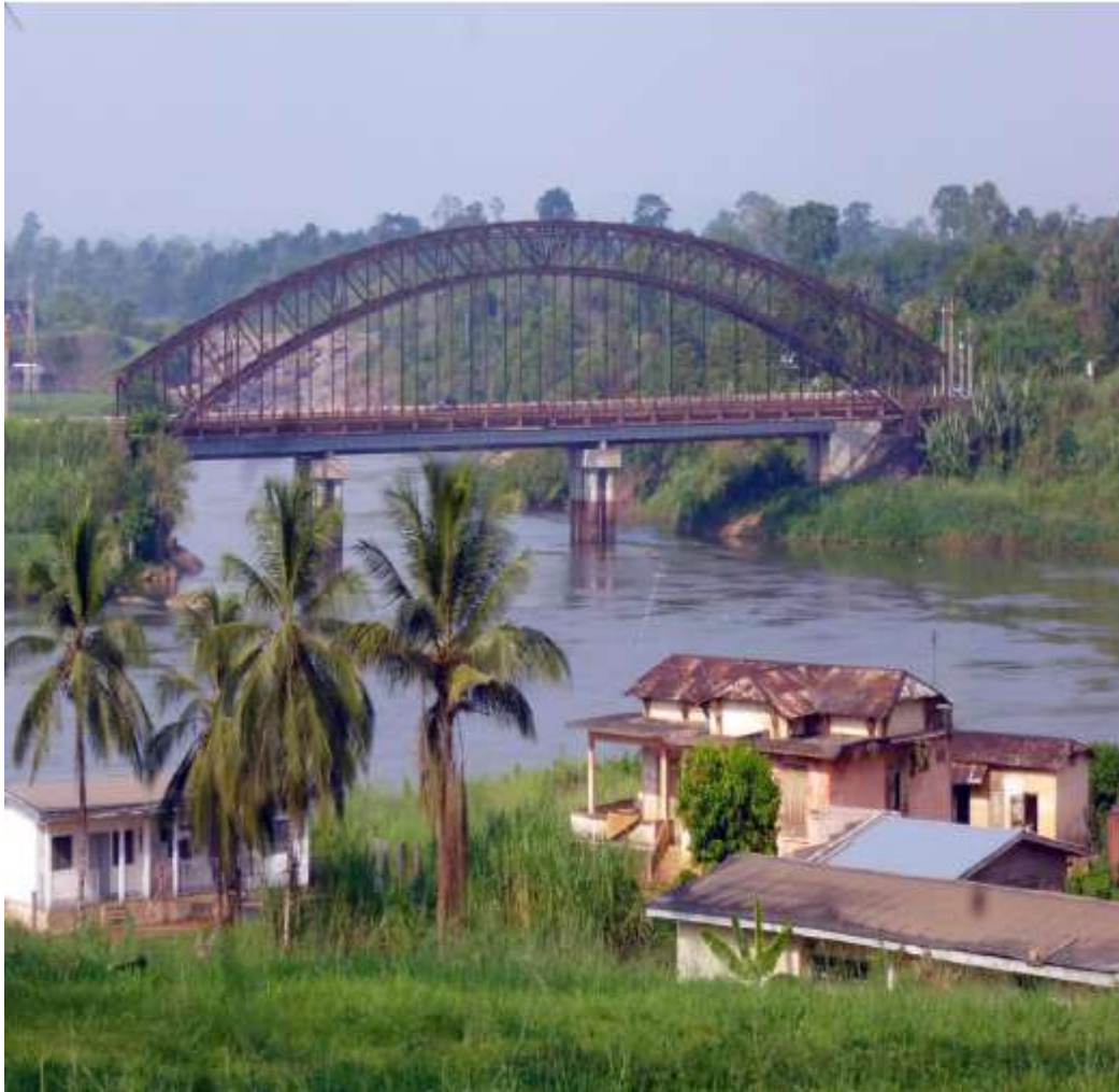
Figure 2: A View of the German Railway Bridge in Edéa
