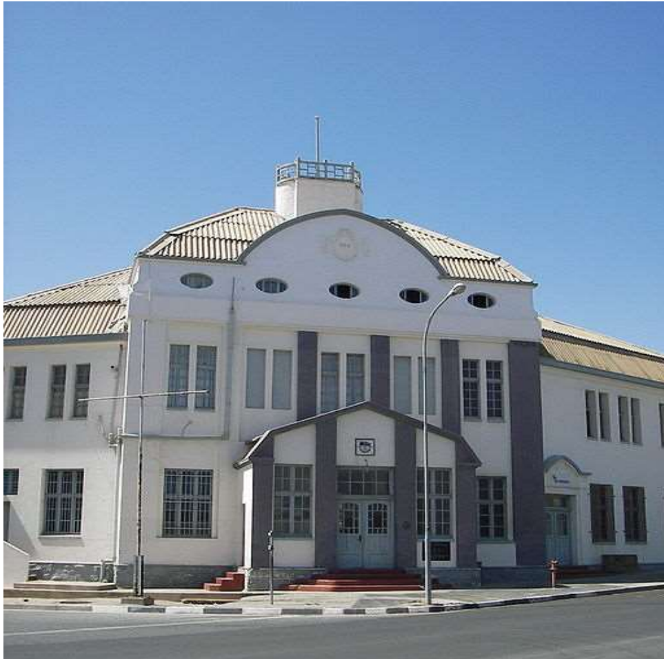
Figure 3 : Main facade of the railway station of Lüderitz Building
