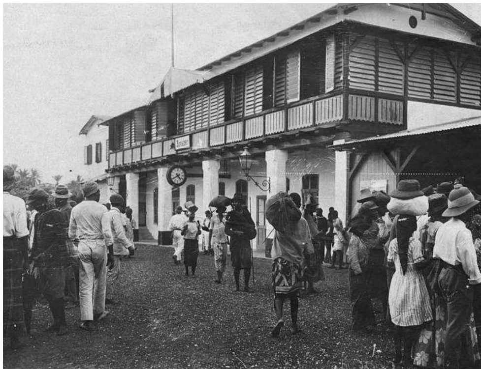
Figure 24 : Nordbahn railway Station, Douala
