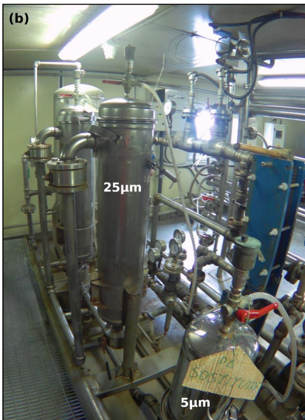
Figure 2: Desalination plant of Mario Zucchelli station. (a) View of the plant pump shed in the locality of Punta Stocchino. (b) 25 \mu\text{m} (left) and 5 \mu\text{m} (right) filter housings in the desalination plant powerhouse. (c) New cartridge filters (5 \mu\text{m} ) just replaced before the closure of the lid of the filter housing. From Cecchetto et al. (2021).
