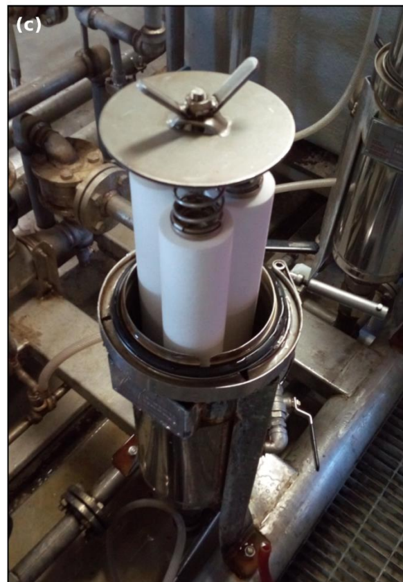
Figure 2: Desalination plant of Mario Zucchelli station. (a) View of the plant pump shed in the locality of Punta Stocchino. (b) 25 \mu\text{m} (left) and 5 \mu\text{m} (right) filter housings in the desalination plant powerhouse. (c) New cartridge filters (5 \mu\text{m} ) just replaced before the closure of the lid of the filter housing. From Cecchetto et al. (2021).
