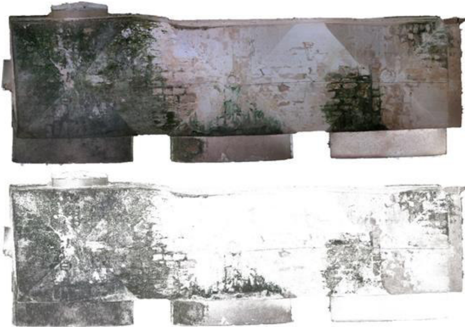
Fig. 46 On the top: Orthophoto of the intrados of the three cross-vaults, below Orthophoto with only green colours extracted
