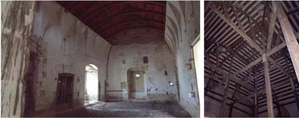
Fig. 76 Current condition of the intervention areas
