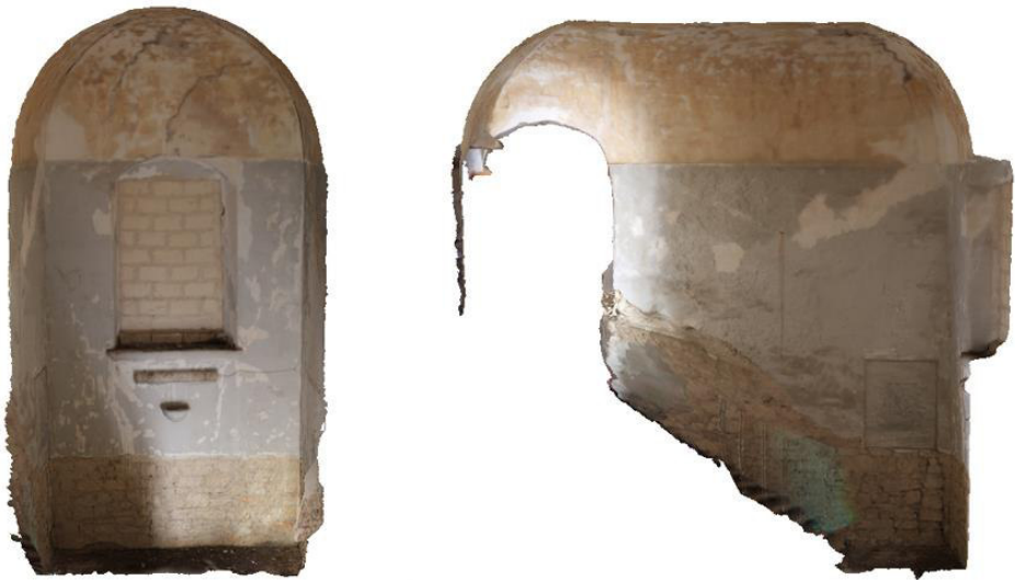
Fig. 90 Portion of dense point cloud of VS02
