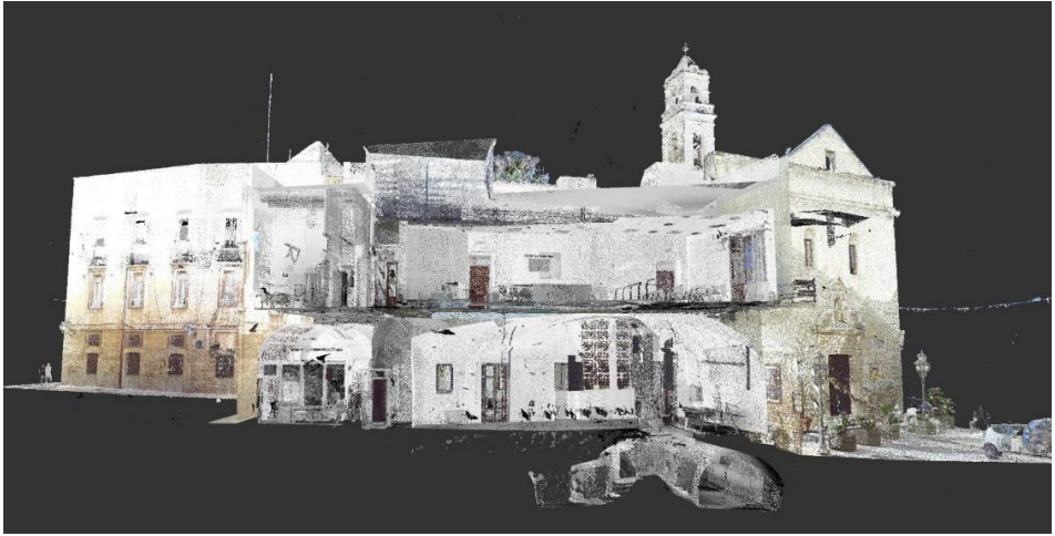
Fig. 24 Section of point cloud of Santa Croce Monastery, Modugno, Italy
