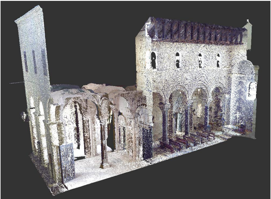
Fig. 25 Section of point cloud portion of Ognissanti Church, Trani, Italy
