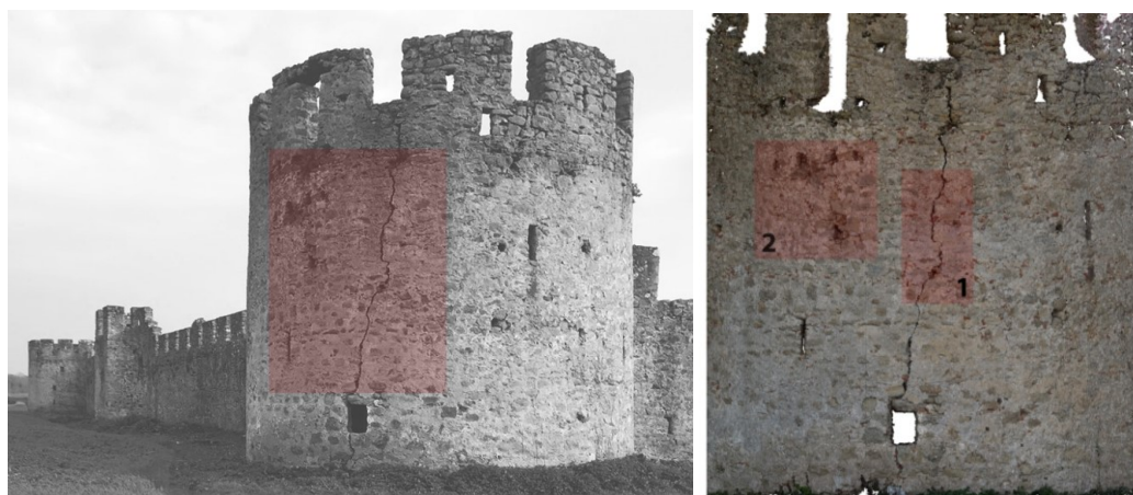
Fig. 52 - North tower of the Fortress of Basthovë. with the indication of samples used for the application of the methodology.
