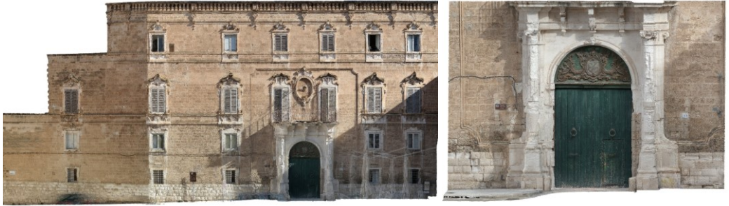
Fig. 33 - High-resolution texturized polygonal mesh of the main façade, with a zoom on the portal [4],[16].
