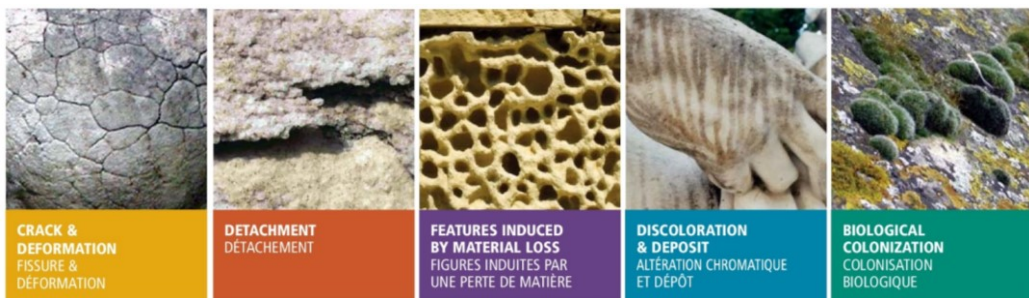
Fig. 8 – Five macro-areas of surface alteration, identified by ICOMOS ([28])
