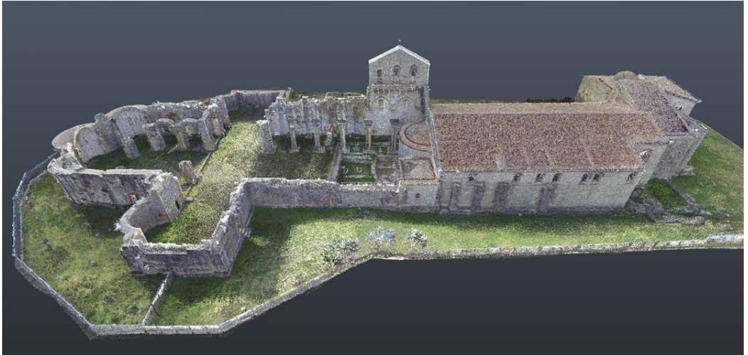
Fig. 47 Integrated point cloud of the entire complex.
