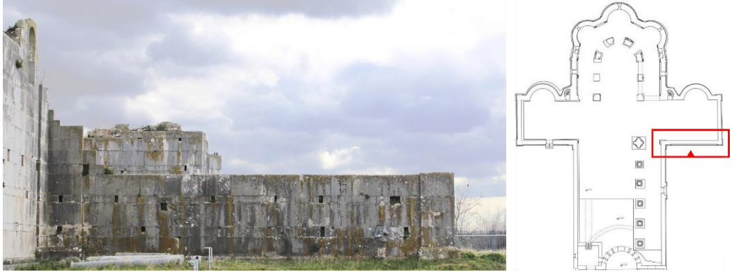
Fig. 51 Southwest façade of the Unfinished Church.
