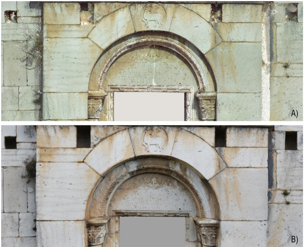
Fig. 49 Comparing 3D polygonal models of the 'Unfinished' church portal: A) range-based method; B) image-based method.
