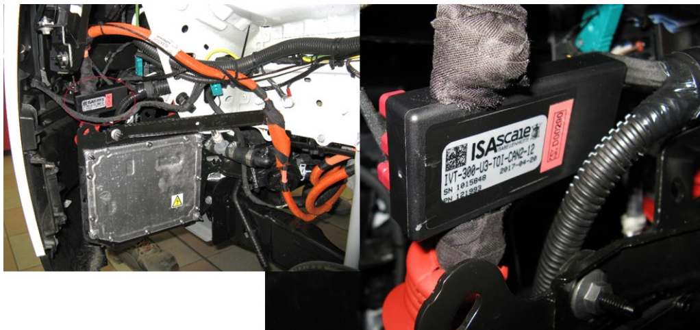
Figure 16: Shunt installation on the DC/DC HV side
