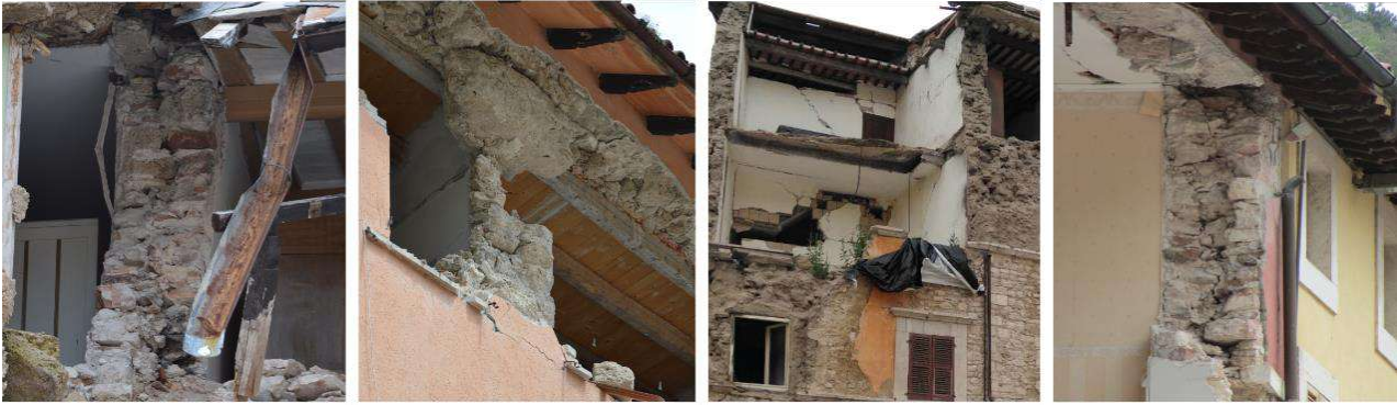
Figure 2. Example of walls and floors visible in other buildings of the historic center of Visso.
