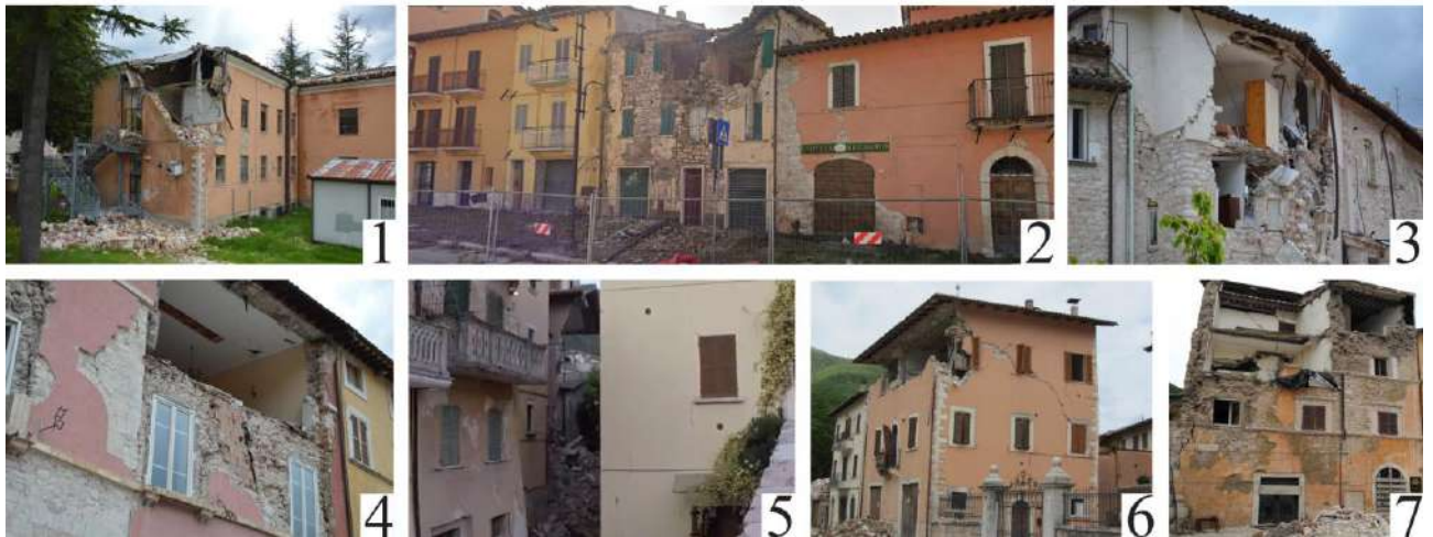
Figure 5.15. Experimental evidence on the OOP occurrence in Visso's municipality after the Central Italy earthquake.
