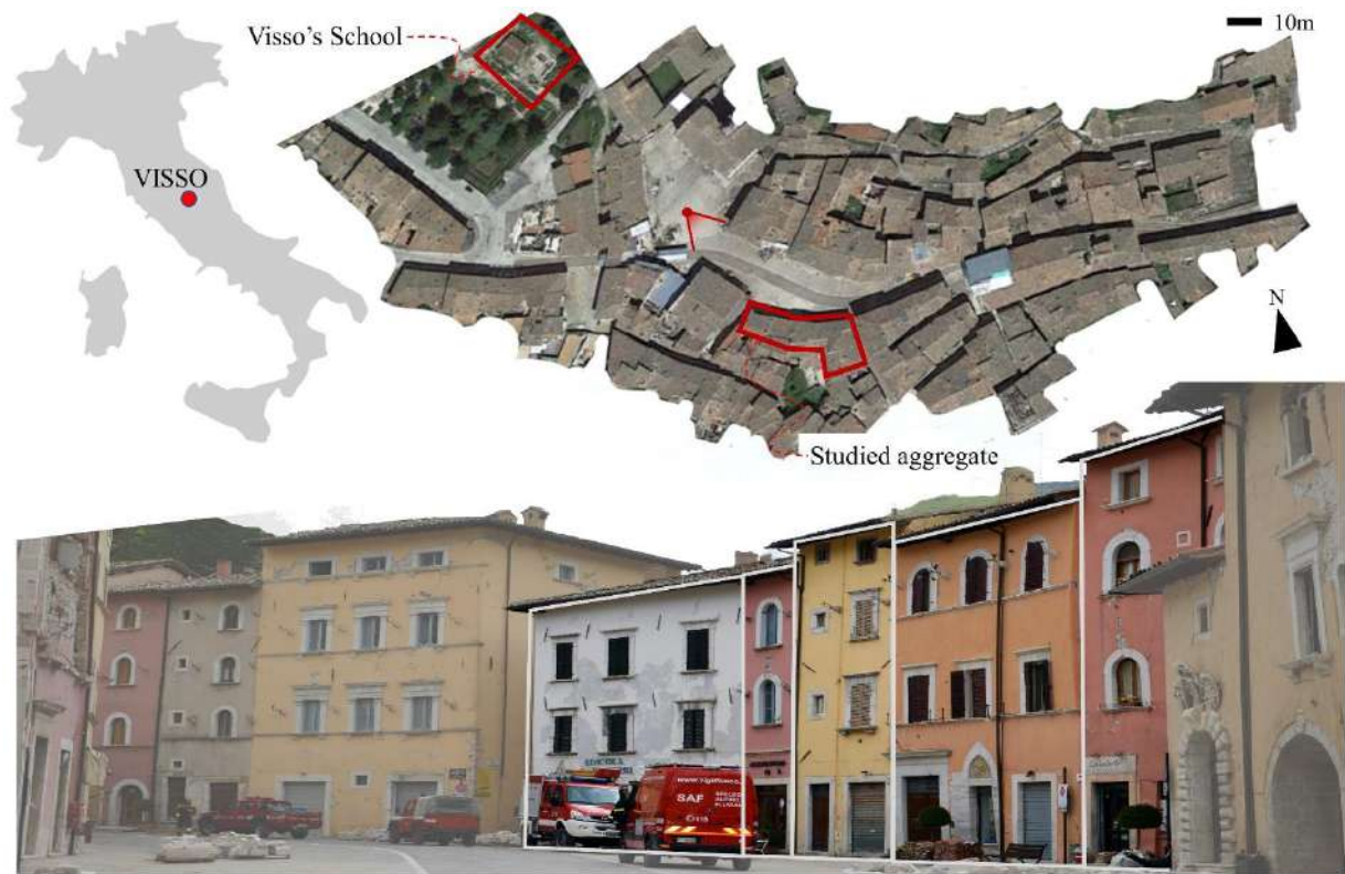
Figure 4.2.2. The case study aggregate in the historical centre of Visso with the indication of the five structural units in the façades facing the municipality's square (U1 to U5 from right to left; picture bottom).
