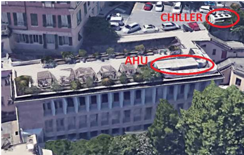
Figure 3.23: Top view of the test site, with AHU and Chiller (©2018 Google)
