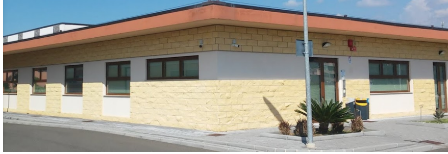
Figure 3.17: Technological pole building.
