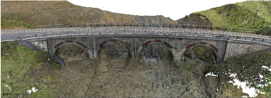
Figure 27 - Point cloud obtained through UAV survey
