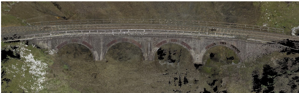
Figure 26 - Point cloud obtained through TLS survey
