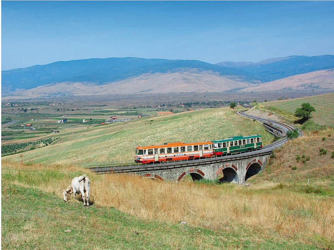
Figure 3 - One of the Circumetnea's lava stone bridges in Maletto (CT) – Ref: Circumetnea archive
