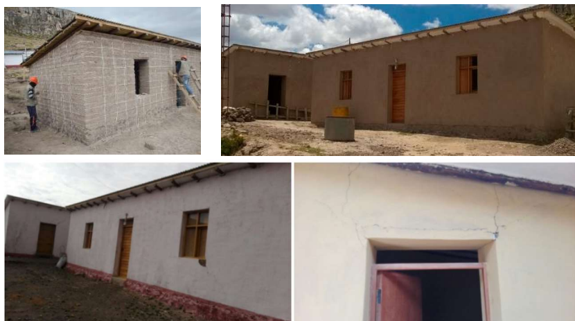
Figure 18 – The upper images show the use of nylon ropes reinforcements in Lampa buildings by the Centro Tierra PUCP [175], the lower images show the minimal damages suffered after the 6.3 earthquake of 2016 [images by Rene Cayo].
