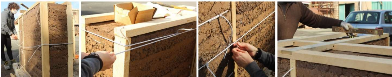
Figure 37 – Full scale prototype construction phases (F-I).
