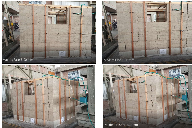
Figure 17 - Lack of connections between the timber post and the walls with issues at the corner [147] (Eng. Urbano Tejada Schmidt).
