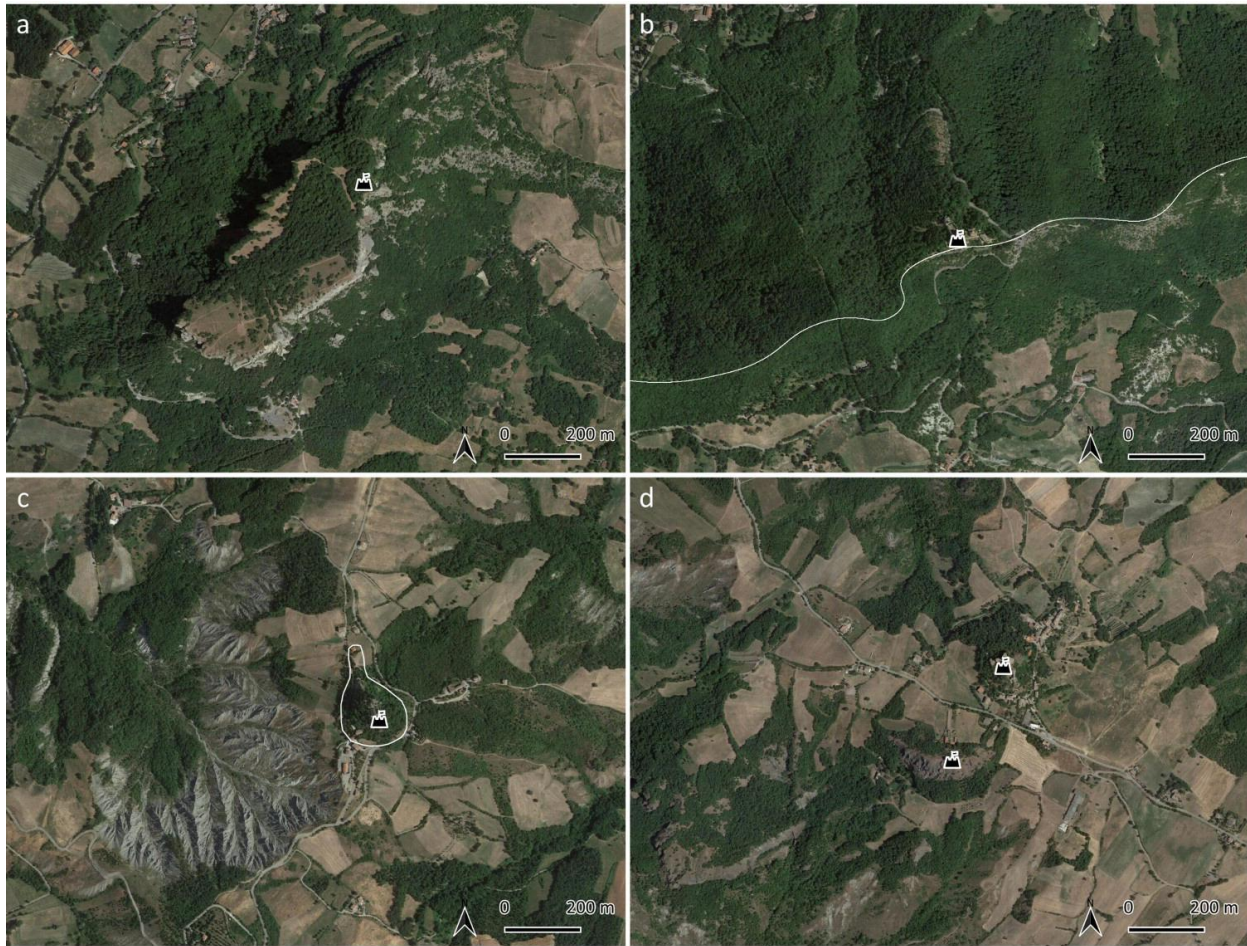
Figure 3. Examples of geological and geomorphological settings of selected castles (satellite imageries from GoogleEarth™): (a) the Pietra di Bismantova castle on top of a mesa-type relief; (b) the Carpineti castle on the rim of a monocline structure; (c) the Canossa Castle on a residual hill of sandstone surrounded by badlands developed on marls and clays; (d) the Guardiola (bottom) and Rossena (top) castles built on top of ophiolite domes.
