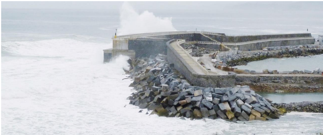
Figure III.12 OWC plant installed in the bay of Mutriku (Spain) [160]
