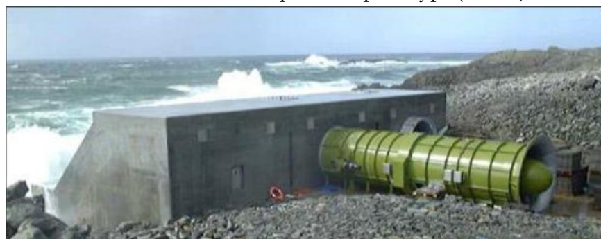
Figure III.10 LIMPET OWC plant installed on the island of Islay (Scotland, UK) [158] (Elsevier license n. 4707221496823)
