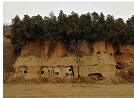
Figure 25. Abandoned house caves ( yaodong ) in Doujiabu Village. © Y. OU (2018)
