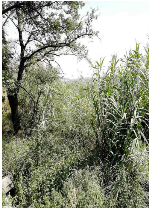
Figure 71. Poorly managed drainage ditch shared by several olive grove owners near Sant'Agata. © Y. OU (2018)
