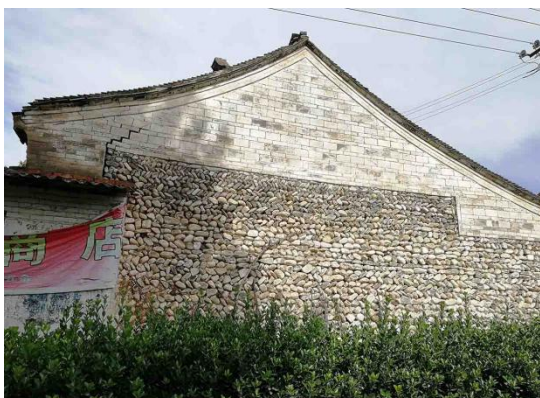
Figure 24. Abandoned construction technique of dry stone walls near Xizhai Village. © Y. OU (2018)
