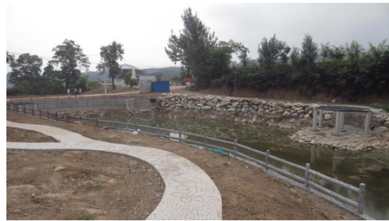
Figure 35. Excessive removal of original vegetation and hardening of pathways of the laochi in Heiyu Village, Meixian County. © Y. OU (2017)
