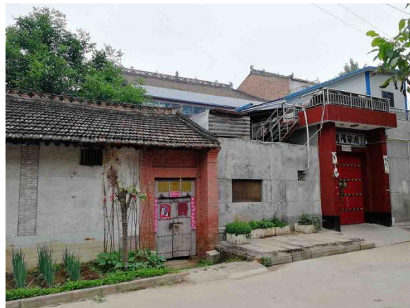
Figure 72. Residents located upstream of the ditch tend to heighten the foundation for better drainage and flood prevention to the detriment of their neighbors (Xiguan Village). © Y. OU (2018)
