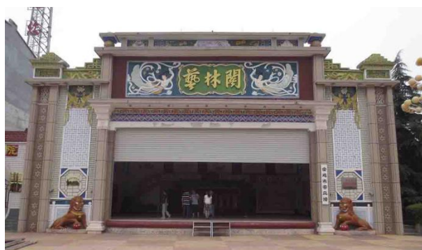
Figure 55. Repurpose of the theater of Hengqu Village as the Hall of Family Ethos. © Y. OU (2018)
