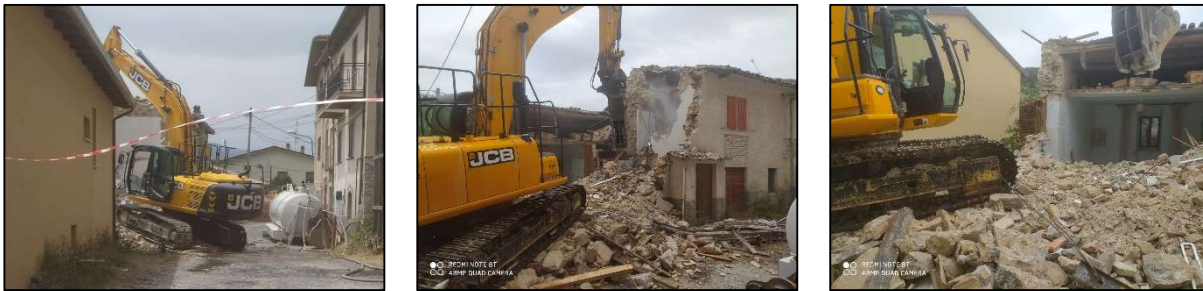
Figure 53: Three different stages of demolition.
