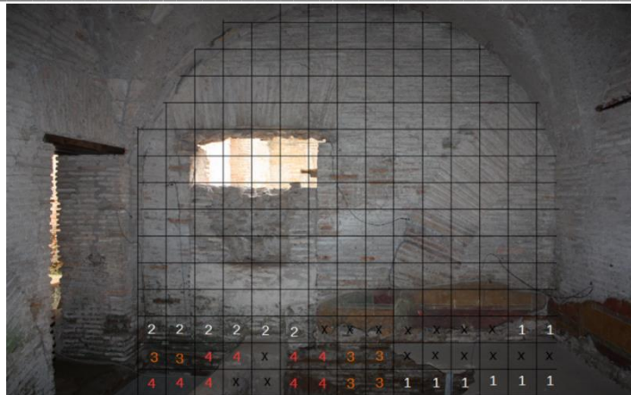
Figure 11. Backside of the investigated wall- Modular grid installation in the Mithraeum room, with the Stage method values assignment. The “x” indicates the frescos presence and so the no value assignment.
