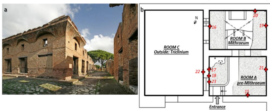
Figure 2. Image of “Casa di Diana” building (a) and plan of measurement strategy (b). The (+) red symbols indicate selected areas in which Raman spectroscopy and HH-ED-XRF analyses were performed.
