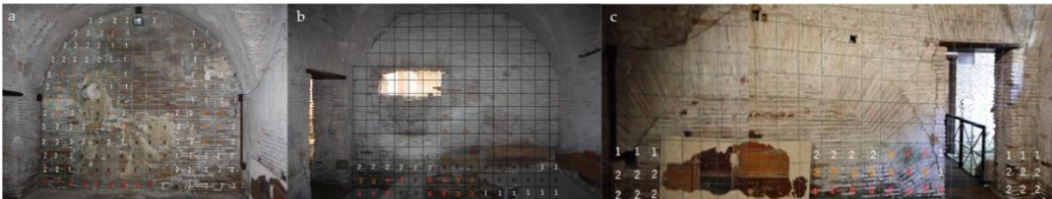
Figure 29. Modular grid installation in pre-Mithraeum room, with the Stage method values assignment. a) East wall; b) west wall; c) south wall.
