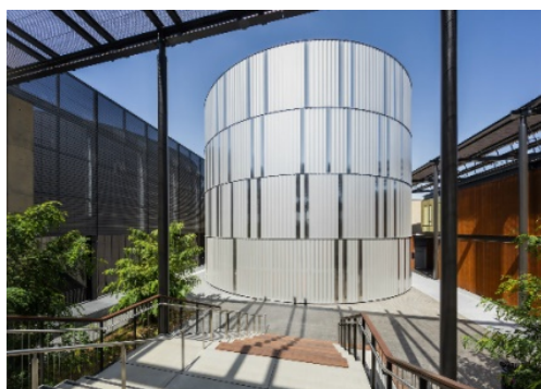
Zgf Architects Llp, Stanford University Central Energy Facility , Palo Alto, California, 2015 Fonte: www.dezeen.com
