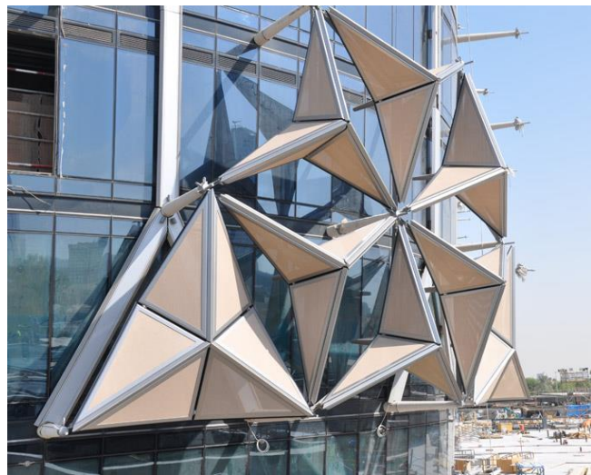
Figure 4.28: Close-up of dynamic façade in folded and unfolded states. Image source: http://www.archiscene.net/firms/aedas/al-bahar-towers/
