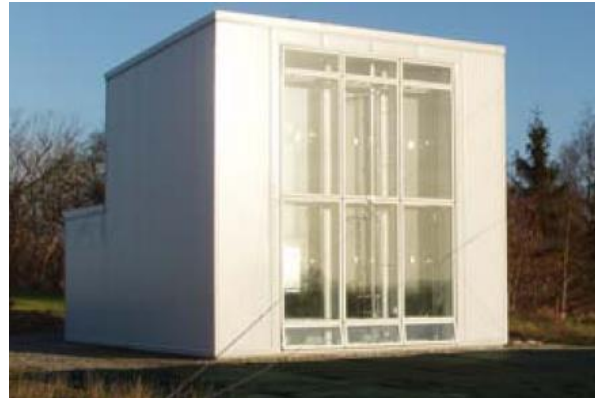
Figure 3.4: The Cube at Aalborg University with a South-facing double façade (Kalyanova, et al., 2009).
