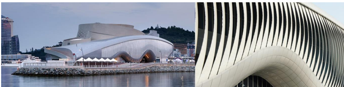
Figure 2.29: Theme Pavilion in South Korea by Soma-Architecture. Left: the main entrance façade to which the biomimetic inspiration was applied in the form of kinetic lamellas that control daylight. Right: close-up of the lamellas in their open position (Soma, 2012).
