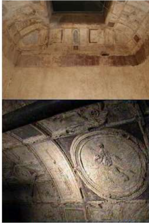
Fig 3 Vestibule cloister vault
