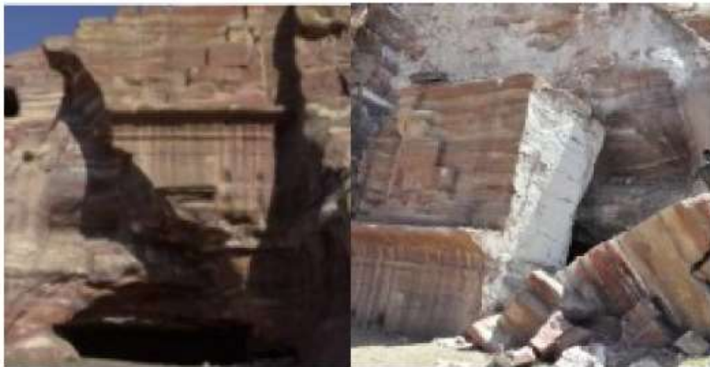
The heartbreaking destruction of monument 609 in Petra by torrential rainfall in early 2010
